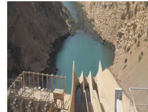
E&I Works- Hydroelectric Central IRAQ –: National Ministry of Energy
