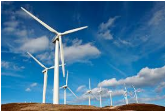
WIND – 9 MW (6x1.5) – TUSCANY Client: GESPI SPA
