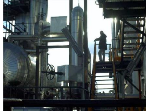
BIOMASS PP- 11 MW – EMILIA Client: San Marco Bioenergie
